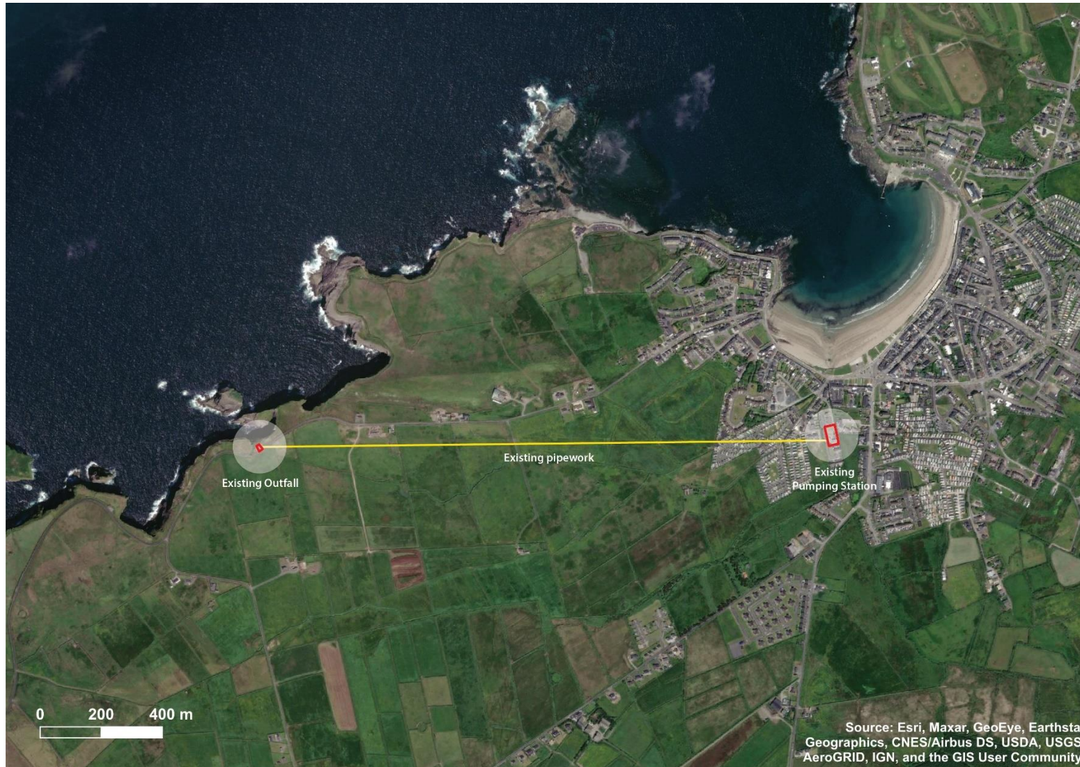
Figure 2: Existing Victoria Park Pumping Station, Existing Outfall and Existing Pipework (Figure 3.1 from Site Selection Report)
